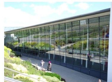
Telford Conference Centre
